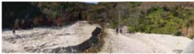
Fig. 17 - Sediment deposition caused by the upstream check dam on the Hachimandani River (View from downstream to upstream direction on December 8, 2009)
