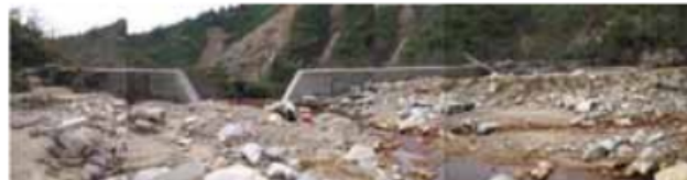
Fig. 6 - Sediment deposition caused by the upstream check dam on the Tsurugi River (View from upstream to downstream direction on November 27, 2009)
