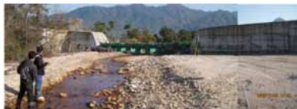
Fig. 23 - Sediment deposition caused by the downstream check dam on the Hachimandani River (View from upstream to downstream direction on November 25, 2009)
